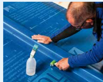
Fig. 18: Welded underlay membrane with enclosed counter batten – this represents the highest category of additional rain-protection measure; it offers very high protection against rain, even at particularly low roof pitches.
