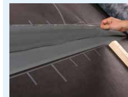
Fig. 41: Membrane overlaps with self-adhesive strips – in this case, the adhesive bond is located under the overlap and is protected against water run-off. The adhesive-to-adhesive bond is reliable even under unfavourable conditions.
