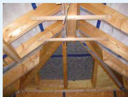
Fig. 31: On this project, monolithic SOLITEX membranes (hip roof at the centre of the photo) and microporous membranes (main roof surfaces on left and right) were installed side by side; under identical conditions, the microporous membrane has a water film, the monolithic membrane remains dry.
