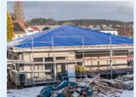
Fig. 2: Tarpaulins covering a roof.
