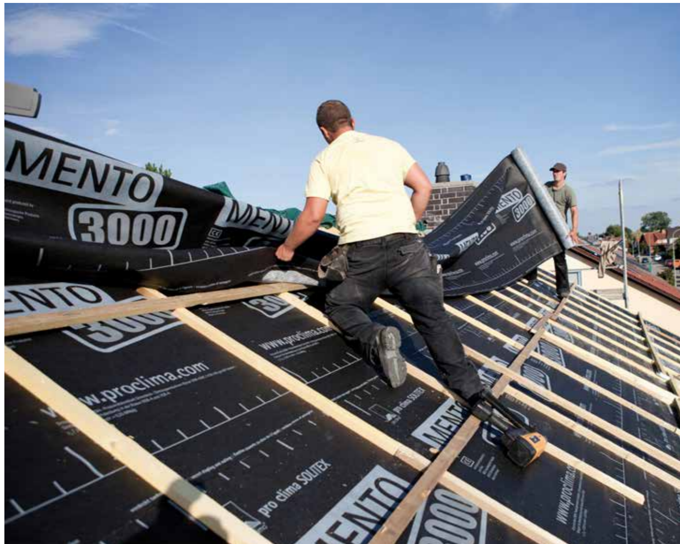
Fig. 1: A modern roofing underlay membrane as an exterior sealing layer underneath the subsequent roof covering.
