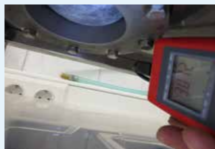
Fig. 38 a/ b: Hydrostatic pressure test after 2 years of natural ageing underneath a roof covering. Top: Microporous membrane leaking at a water column < 0.6 cm; Bottom: SOLITEX MENTO 3000 achieves values > 3 m.
