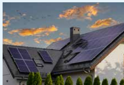
Fig. 8: More demanding conditions may arise due to additional equipment or complicated roof geometries.
