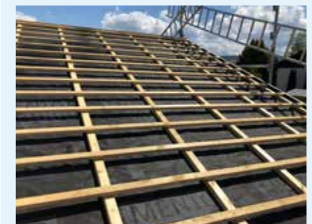
Fig. 4: Roofing underlay with sealed overlaps and joints and with nail-sealing tape (not visible here) to seal perforations.
