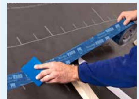
Fig. 5: Obligatory measures when using roofing underlay membranes as a temporary covering: Taping of seams and joints with adhesive tape or integrated self-adhesive strips.
