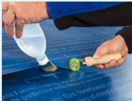
Fig. 20: Welding of underlay membranes: The functional layers of overlapping membranes are welded together homogeneously with a solvent welding agent or a hot air gun.
